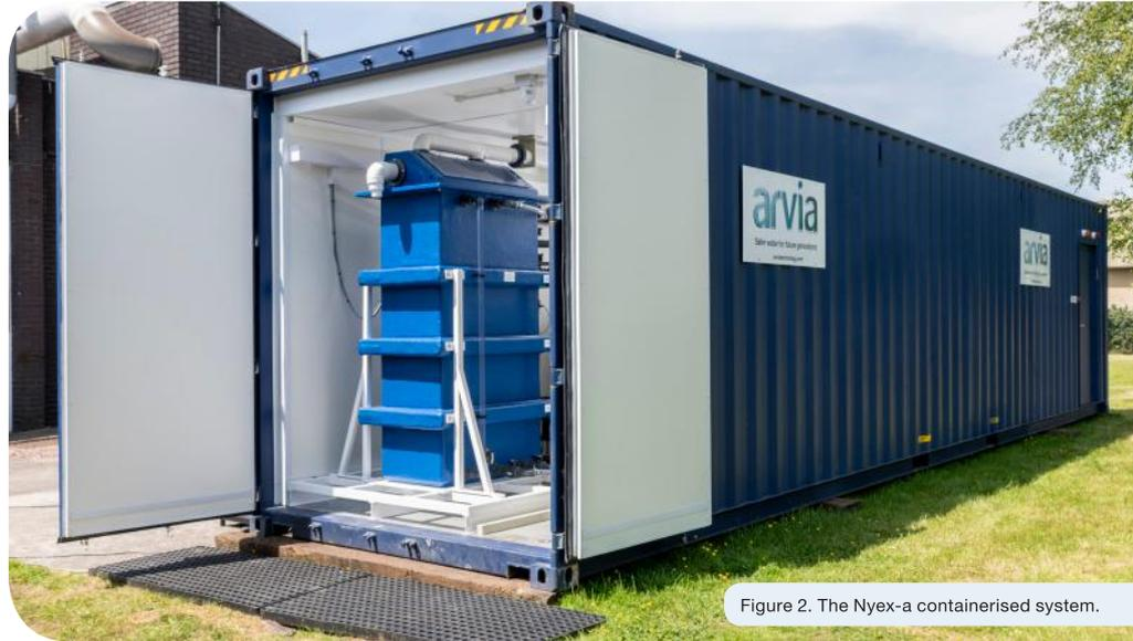
Figure 2. The Nyex-a containerised system.
